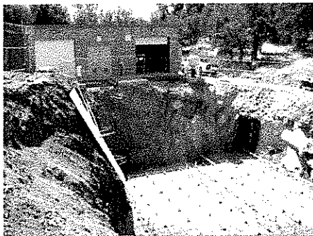
Pump Station Excavation
