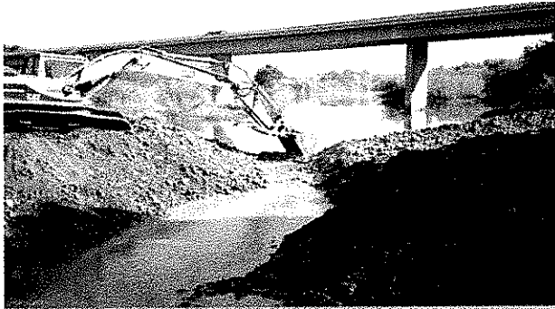
Damming the Tuolumne river to isolate Raw-Water Intake Structure
