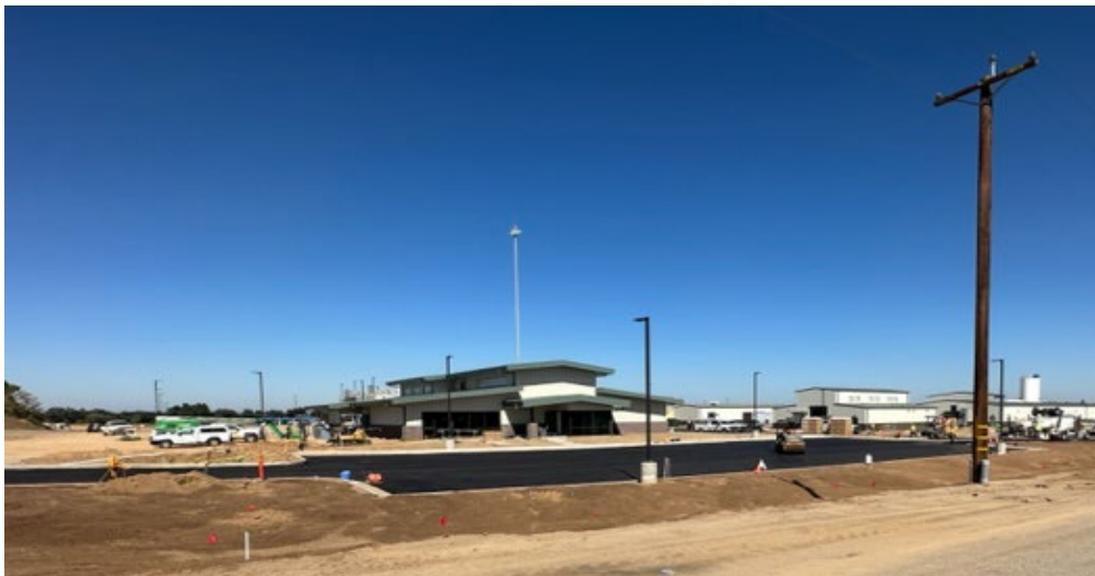
figure 3 - Roads - Asphalt Poured
