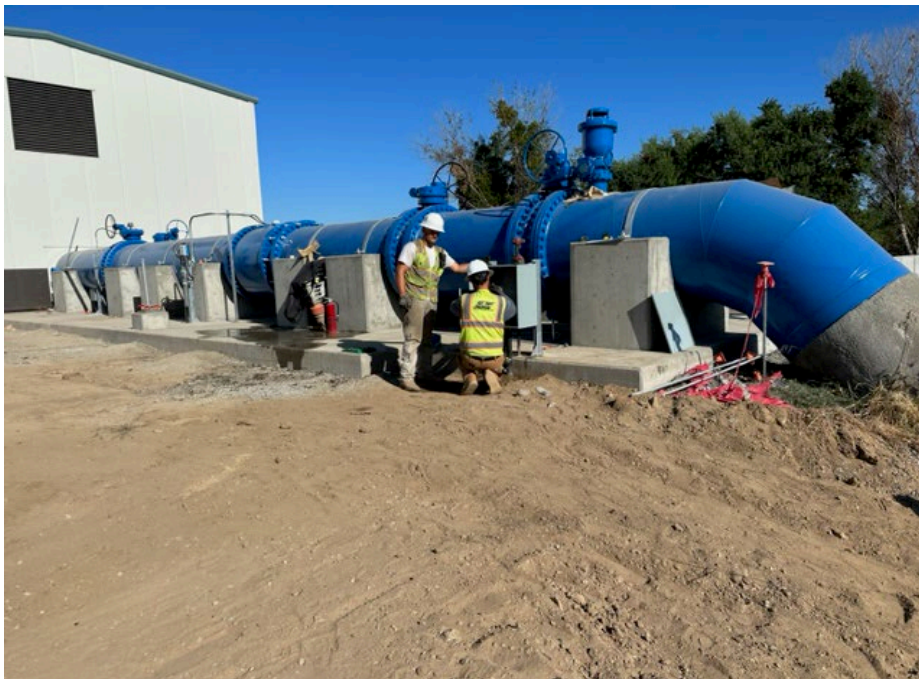
figure 1 - Raw Water Pump Station - Electrical wires landed
