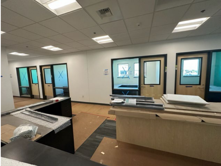
figure 4 - Administration Building - Furniture delivered and installed
